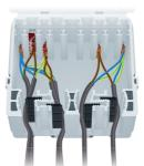
When a single circuit is being supported then cross linking between each side of the enclosure is permitted.
